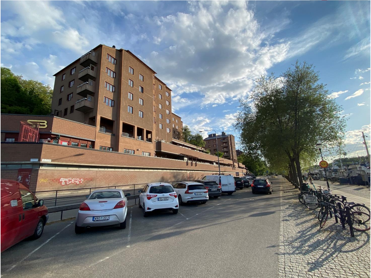
Figure 2 Parking, driveway and closed walls © Alexander Stähle
